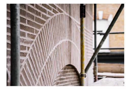
Commence the build of the surrounding brickwork, following local Building Regulation requirements regarding the installation of wall ties around the arch.
