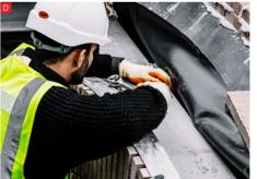
Restrain the arches using the brackets provided by IG Masonry Support at the correct positions.
