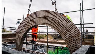
Using approved mechanical lifting equipment, hook up the lifting eyes provided on the arch and crane into position.
