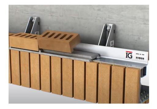
Position compressible filler to underside of horizontal support shelf. Maintain a 2mm space above the filler and install pistol bricks above masonry support shelf.
