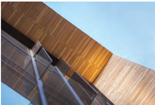
Soffit view of main entrance
