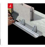
Commence with torquing the masonry support system.
